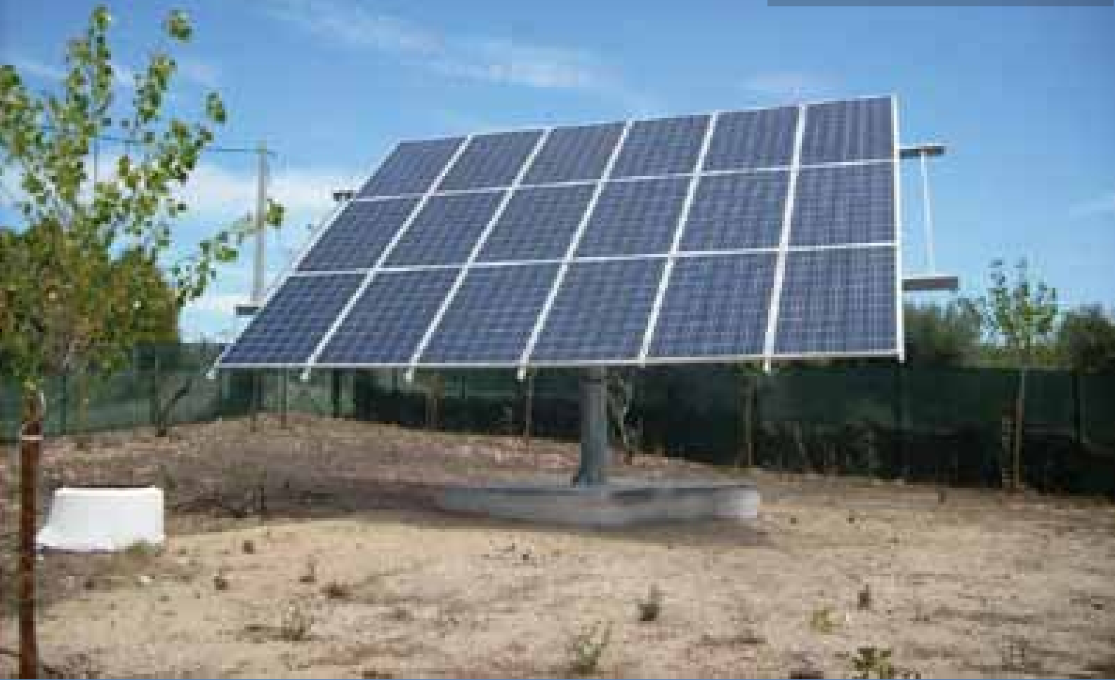
Tripower off-grid, trackers 32 kW
